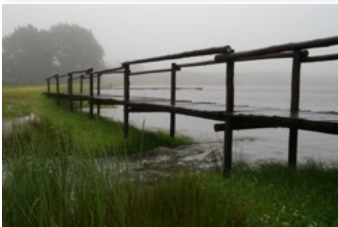
New walkway over Dam 7 Spillway
